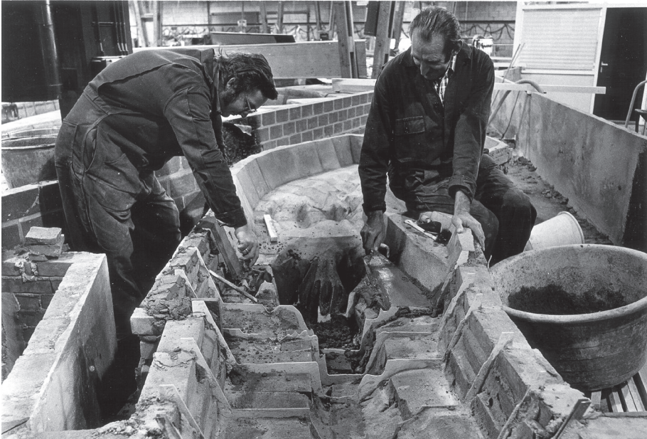
Figure 3.2 The Rijnmond model under construction. © Deltares.
